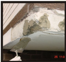
Mortar Repair
