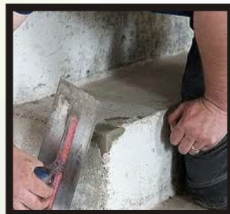
Mortar Repair
