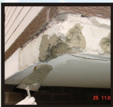
Mortar Repair
