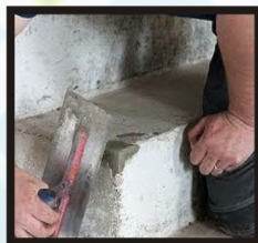
Mortar Repair
